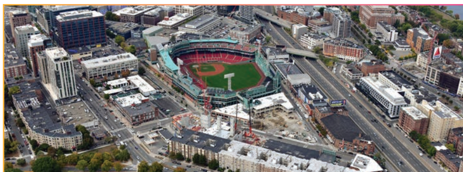
BAA'S NEW SCHOOL BUILDING SITE IN THE FENWAY NEIGHBORHOOD
