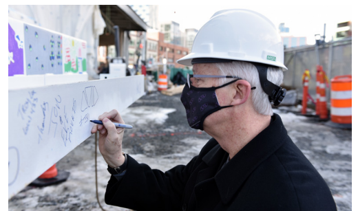
BAA Foundation Board Chairman Jeff Rosica signs the steel beam at the Topping Off ceremony on February 23, 2021.
